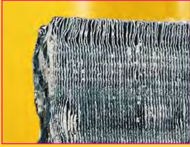
Exposed to Corrosion
